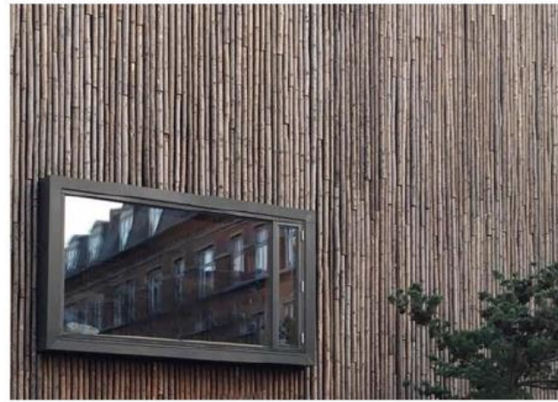
FACADE I RAFTER
